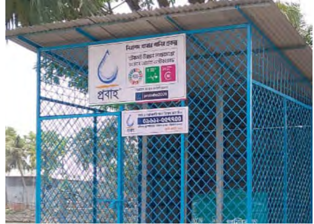
■ 4 new Probaho plants have been installed at Shyamnagar and Assasuni upazila at Satkhira
