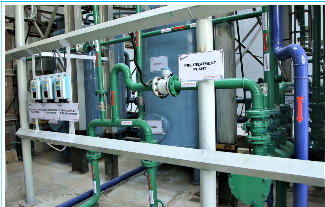
■ Water Line Re-networking at GLTP
